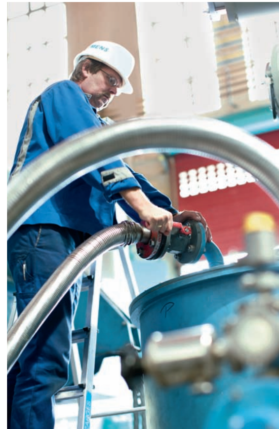
The transformer is being evacuated and filled with insulating oil.
